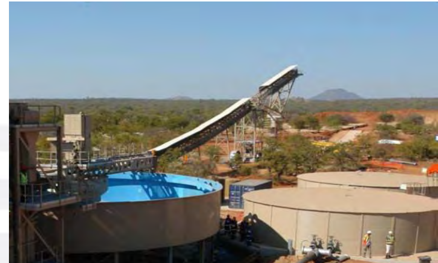
Thickener and product stockpile
